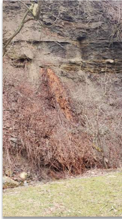
PHOTO 1: Acid mine drainage along WV-88
