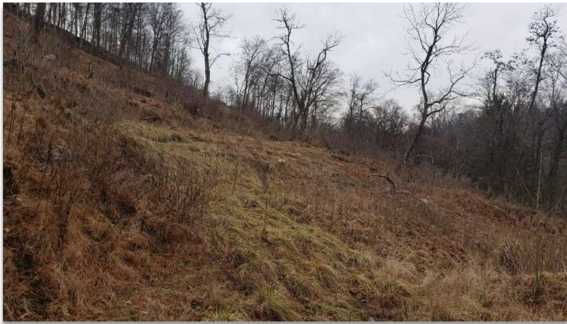
PHOTO 2: Topsoil slide along property
